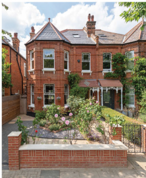
▶ Chevening Road, London NW6. This semi-detached Victorian house has been refurbished to include a dining kitchen extension with self-cleaning solar reflective glass skylights, a temperature-controlled wine cellar, and a parking area with an EV charging point. 5 beds, 3 baths, dining kitchen, dressing room, recep, office/playroom, garden studio with en-suite bathroom, garden. £4.25m Knight Frank 020-3815 3020.
